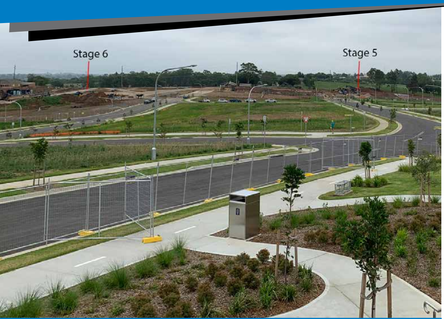
Above: The view from Caddens Hilltop Park - Stage 5 (right) has recently been registered with LRS with Stage 6 (left) under construction Top right: Basketball courts in the new Caddens Hill Sports Precinct Bottom right: Open day at Caddens Hilltop Park.
